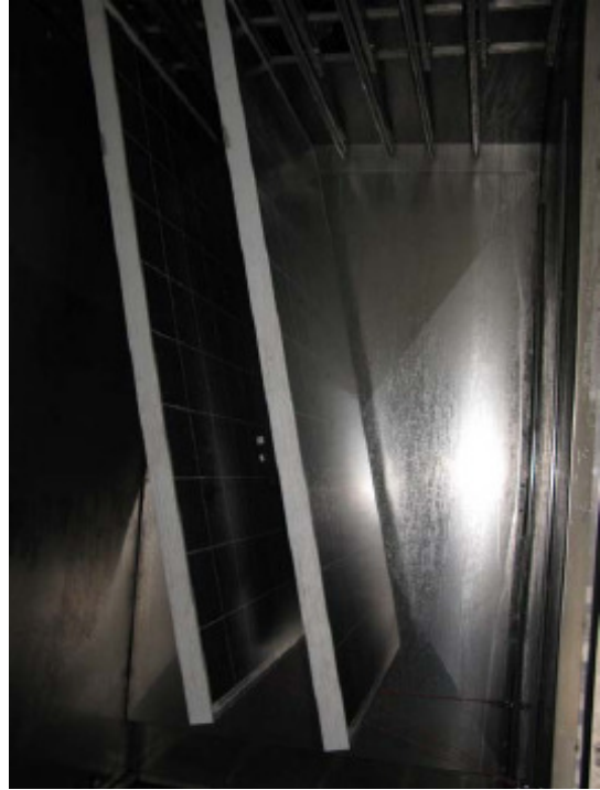
After ammonia test
